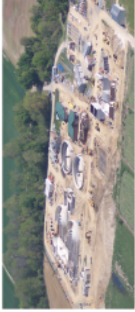
Easton Utilities Enhanced Nutrient Removal Wastewater Treatment Facility under construction
